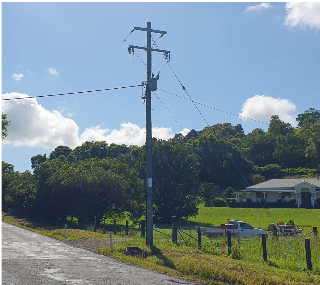
Figure 5: Extent of the overhead 11kV network and pole substation, north of the site (not 3-phase)
